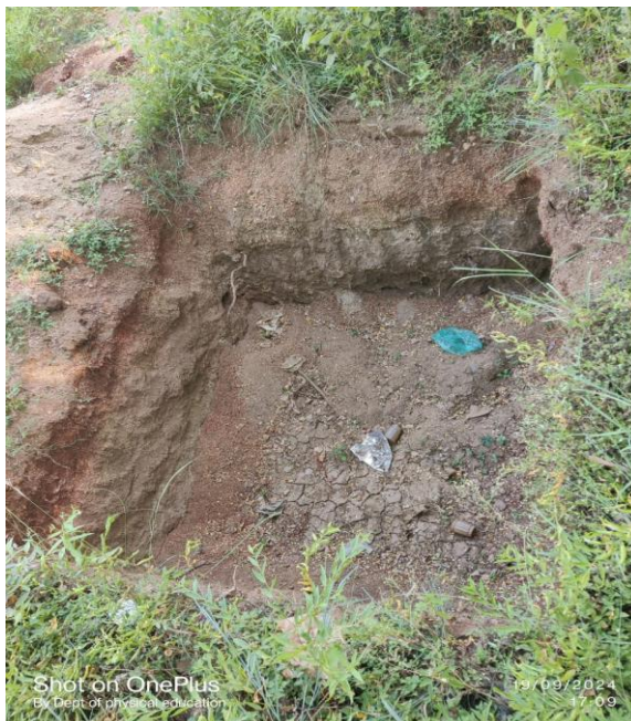
Two more rain water harvesting pits under construction
